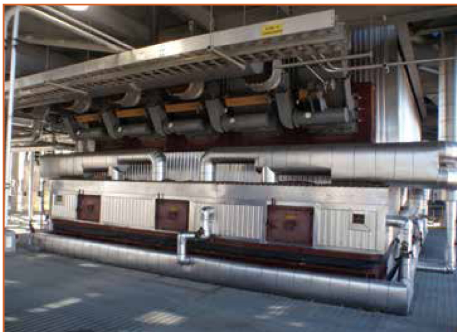
Grate system and fuel distributors
